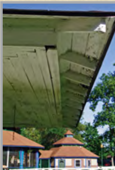
Left photo: Deteriorated soffit was replaced. Right photo: SERVE Noblesville volunteers painted the building
